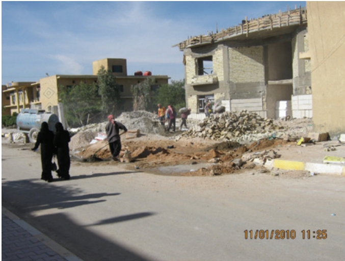
Figure 1: construction site at Karbala University (old campus)
