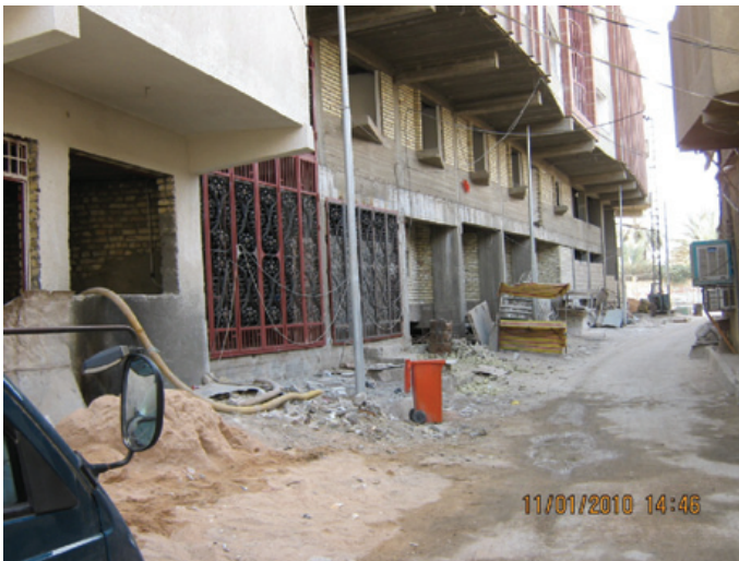
Figure 2: construction site near Karbala city centre
